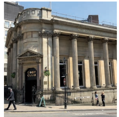
The Birmingham Banking Company building
